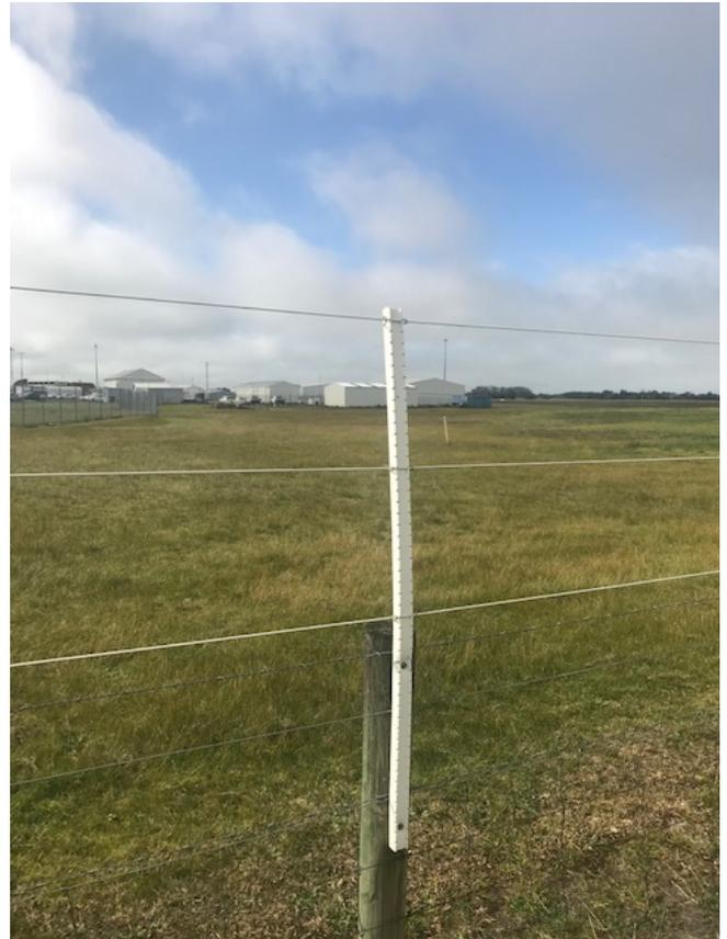
Photo: Mt Gambier airport's fence, showing the white dropper extension to deter kangaroos – supplied
