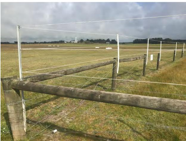
*Photo: the white poly droppers and sighter wire in place*
